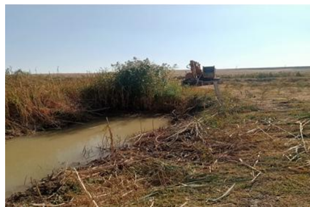
Figure 3. Zhanaaryk drainage collector affected by siltation and vegetation overgrowth, Saryagash district
