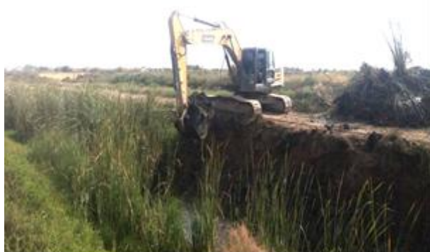
Figure 1. Mechanical cleaning of an overgrown drainage collector using an excavator
