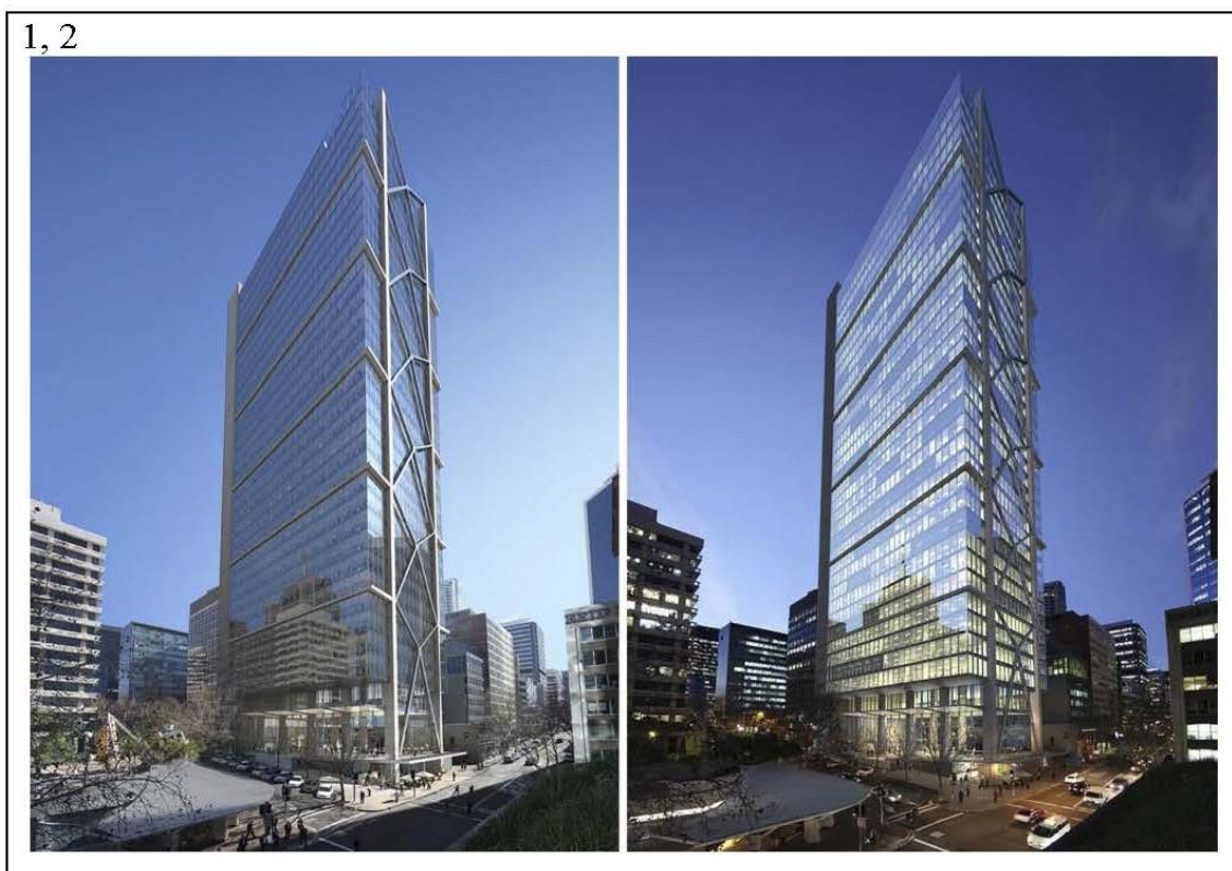
Figure 12. 1, 2. Commercial building, Sydney, Australia, "SOM", 2019 [8].
