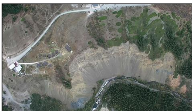
Figure 5. Portside (picture from UAV)
