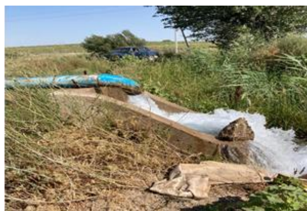
Figure 4. Water discharge into the Eastern «Kazakhstan» collector, Shardara district
