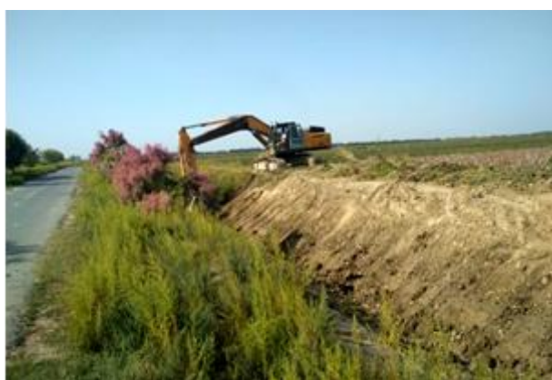
Figure 2. Mechanical cleaning and restoration of a drainage collector
